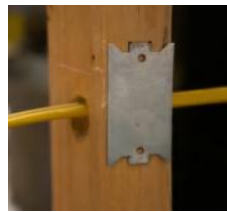
long steel cable protection plate with wood spike for easy hammer on installation on wood studs
