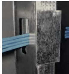
long steel cable protection plate with "peel and stick" adhesive backing for application on metal studs
