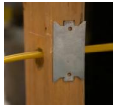
long steel cable protection plate with wood spike for easy hammer on installation on wood studs
